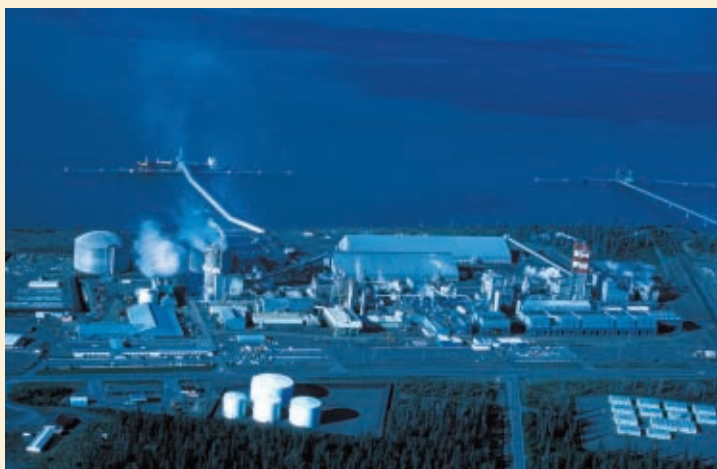
▲ Today, ammonia is produced on an industrial scale in plants like this one.
